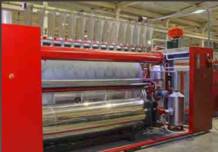
Gas heating system
